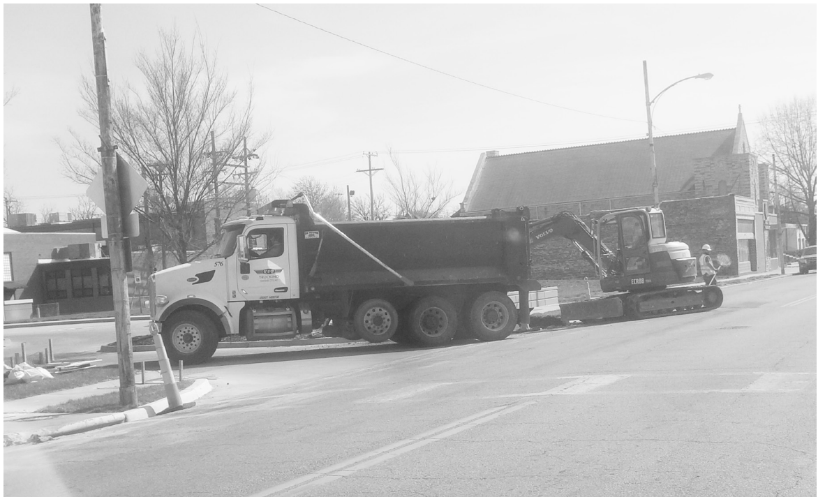
Men doing work on Strong Avenue In Argentine.
