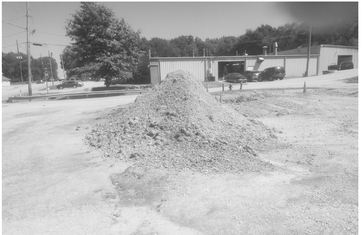
At 49th and Metropolitan, this is all that is left of the place that used to have a reputation. This pile of dirt/gravel is all that is left of the "joint" that used to be Cedar Lawn. Later it was called, "Mind Your Own Business."
